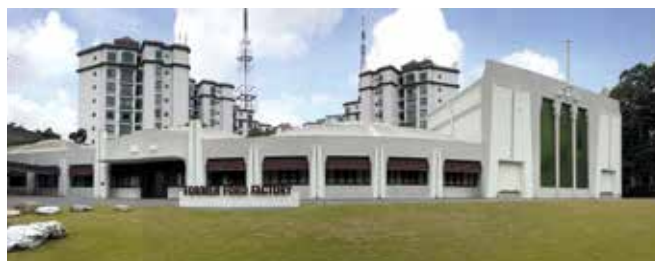
The Ford Factory as it stands today on Bukit Timah Road. The museum preserved façade, with apartment buildings and the radio tower at the back
